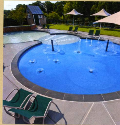
Lothorian Pools , Phoenix, MD Recreation/Leisure
